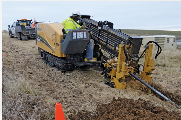
Horizontal Directional Drilling
